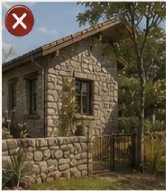
KEYED STONE MASONRY WALL
