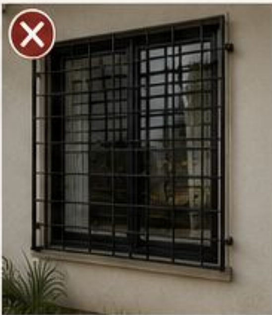
VISIBLE BURGLAR PROOFING
